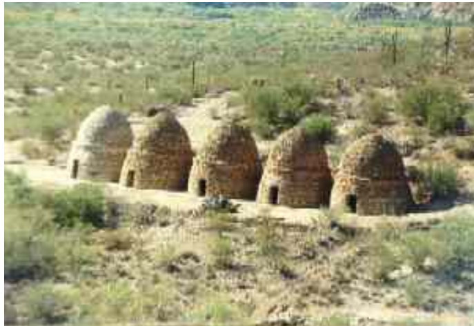
Coke Ovens by Cochran
